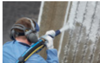
8.6 to 10 bar: Abrasive blasting
